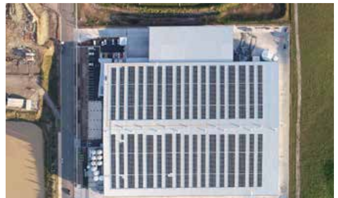
1519 kW onsite solar PV capacity at Horsley Park, New South Wales, Australia
